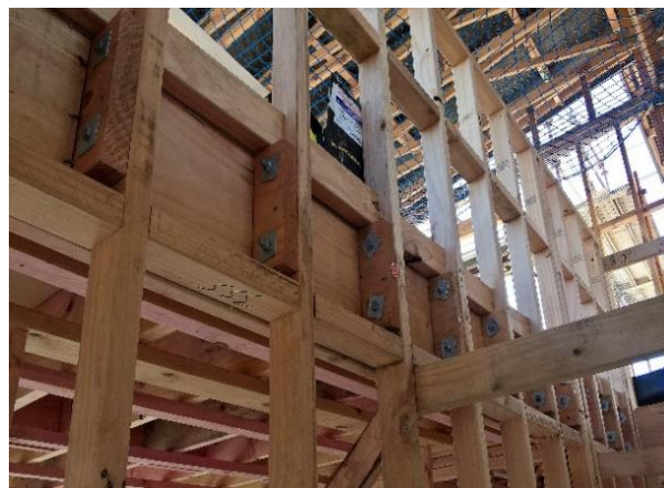
Engineering fixings midfloor joists also see safety net under trusses
