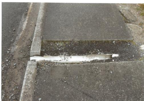
Health and safety – exposed stormwater drain
